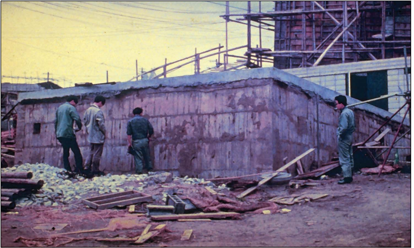
Figure 99: Floating Tank. During a 1964 earthquake in Niigata (NEE-gat-ah), Japan, the ground turned to a dense liquidlike substance, causing this empty concrete tank to float up from just below ground level. This was the first time geologists identified the phenomenon of liquefaction , which had undoubtedly occurred in other large earthquakes. Liquefaction has even lifted empty tanks up through asphalt pavement 1 and raised pipelines and logs out of the ground. 2 In other words, buried objects less dense than surrounding soil rise buoyantly when that soil liquefies. What causes liquefaction? What would happen to buried animals and plants in temporarily liquefied sediments?
