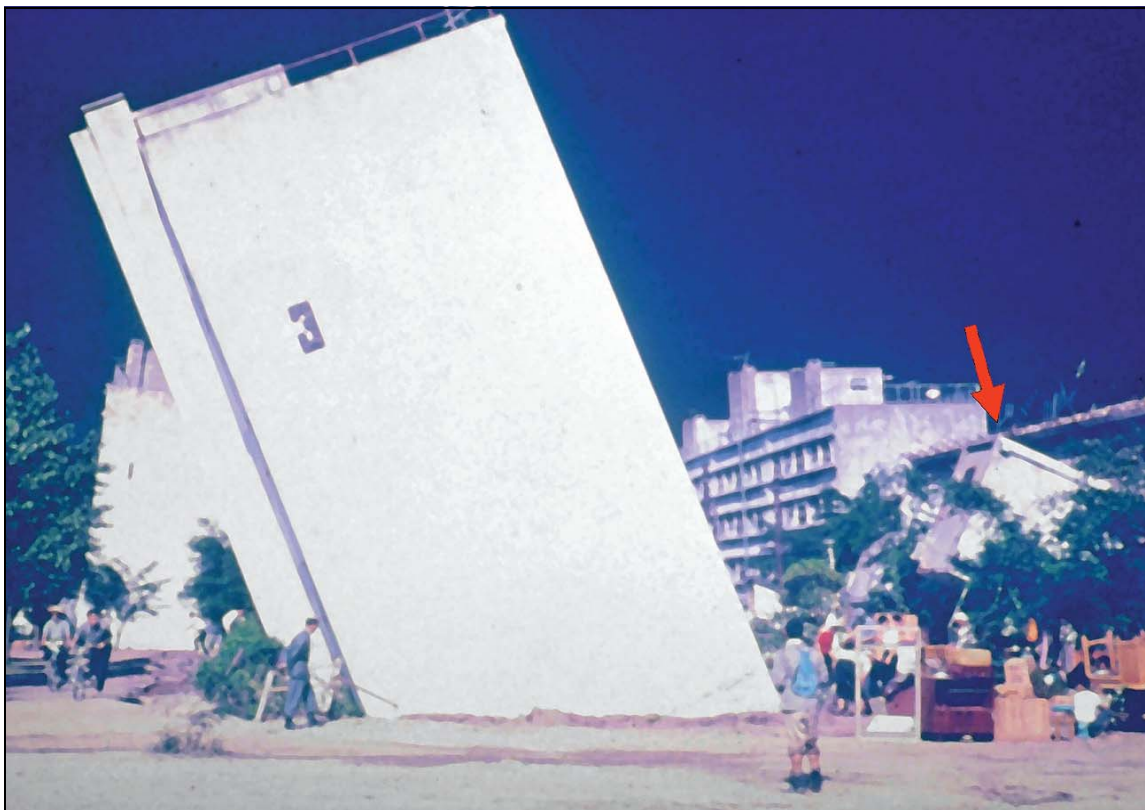
Figure 100: Sinking Buildings. During the above earthquake, building number 3 sank and tipped 22 degrees as the ground partially liquefied. Another building, seen at the red arrow, tipped almost 70 degrees, making its roof nearly vertical.
